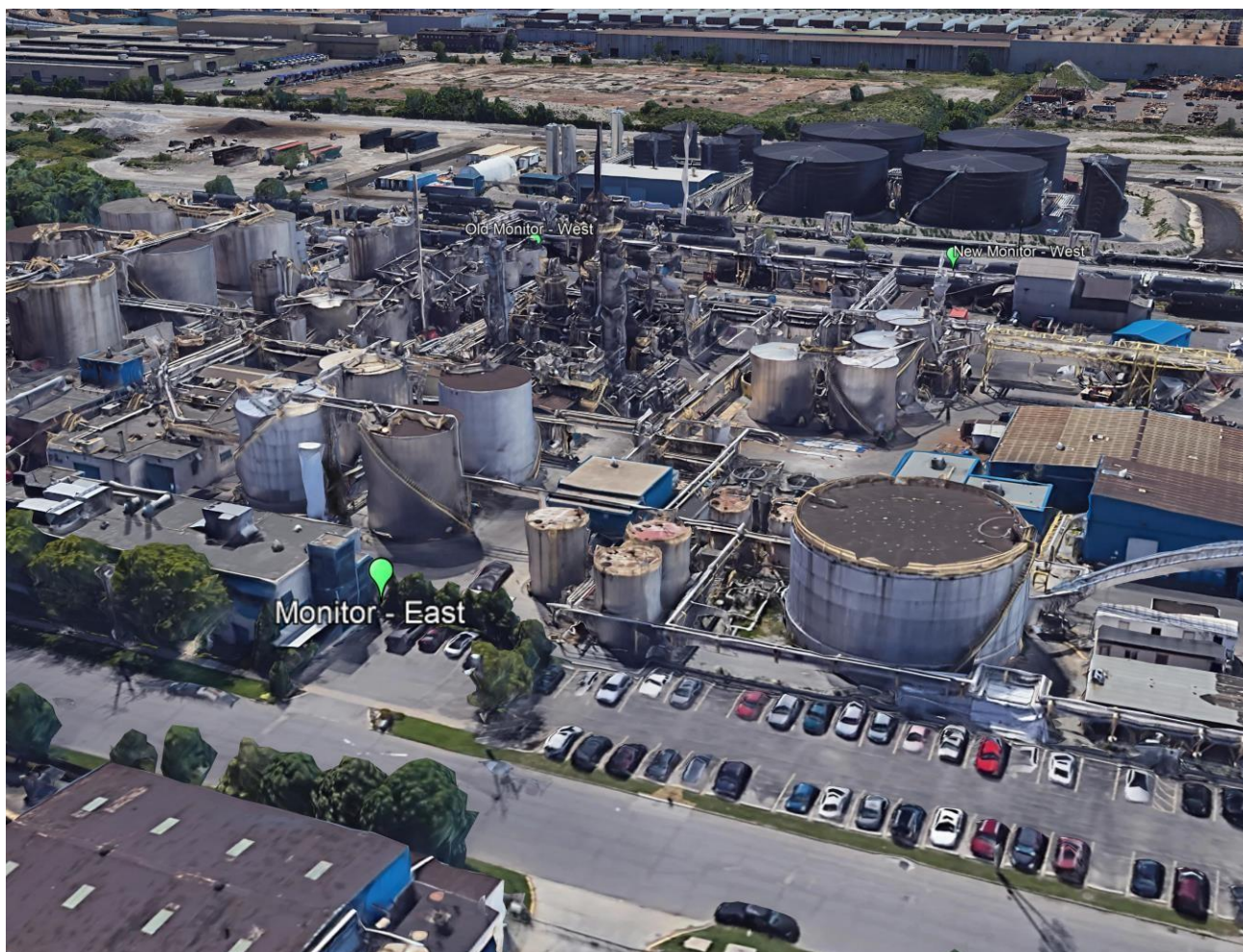
Figure A4: Aerial View 4 – East Monitoring Station
