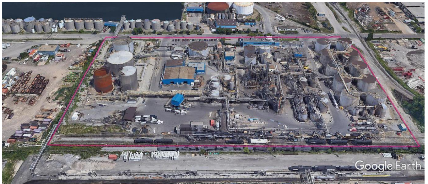
Figure A2: Site-Wide Aerial View 2
