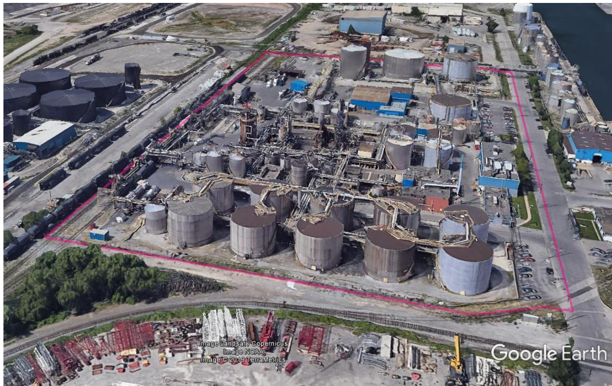
Figure A1: Site-Wide Aerial View 1
